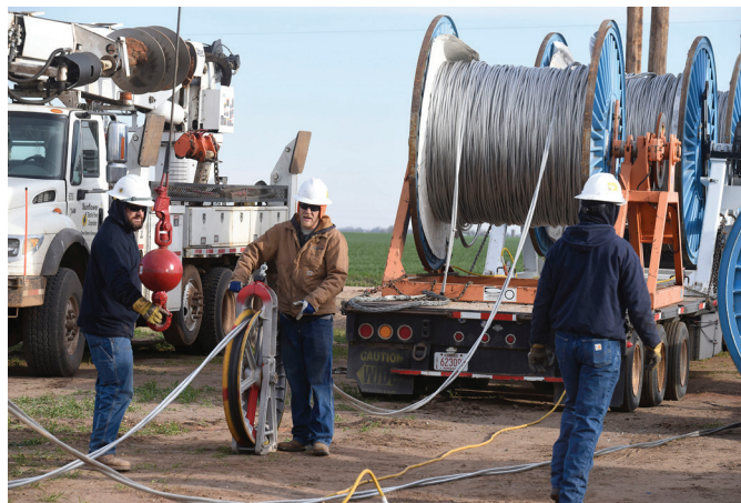
Sunflower employees Michael Creamer, Line Technician Apprentice II, Derek Gilsdorf, Journey Line Technician, and Shane Wheeler, Journey Line Technician, string conductor for the transmission project.
