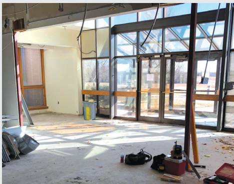
The removal of walls opens up the lobby of the KEC headquarters. Photo taken by Larry Detwiler and Stacey Marston on Jan. 2, 2018.
